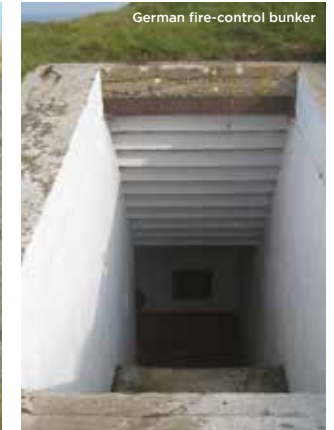
German fire-control bunker
