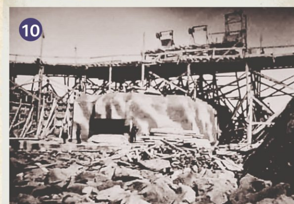
The defences under construction at Bibette Head in 1943, showing the completed 10.5cm casemate.
